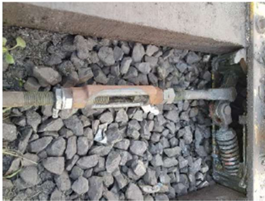
Turnbuckle for rail track HLN M30 SS400 & M30 Left handed * to ensure strengthen the track so that the rails are held in position
